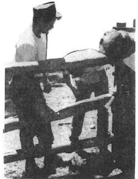
Corral fences needed repair, replacement and reinforcement. New gates were made.
